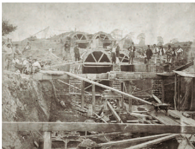
ABOVE: Northern outfall sewer and overflow into the River Lea
